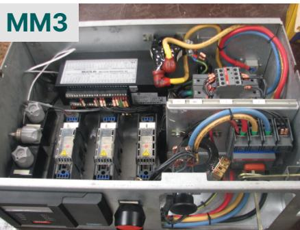
Once the MM3 unit is removed, a supporting plate is installed in the chassis using the existing MM3 mounting holes. A DIN rail is then installed to support the MM300
